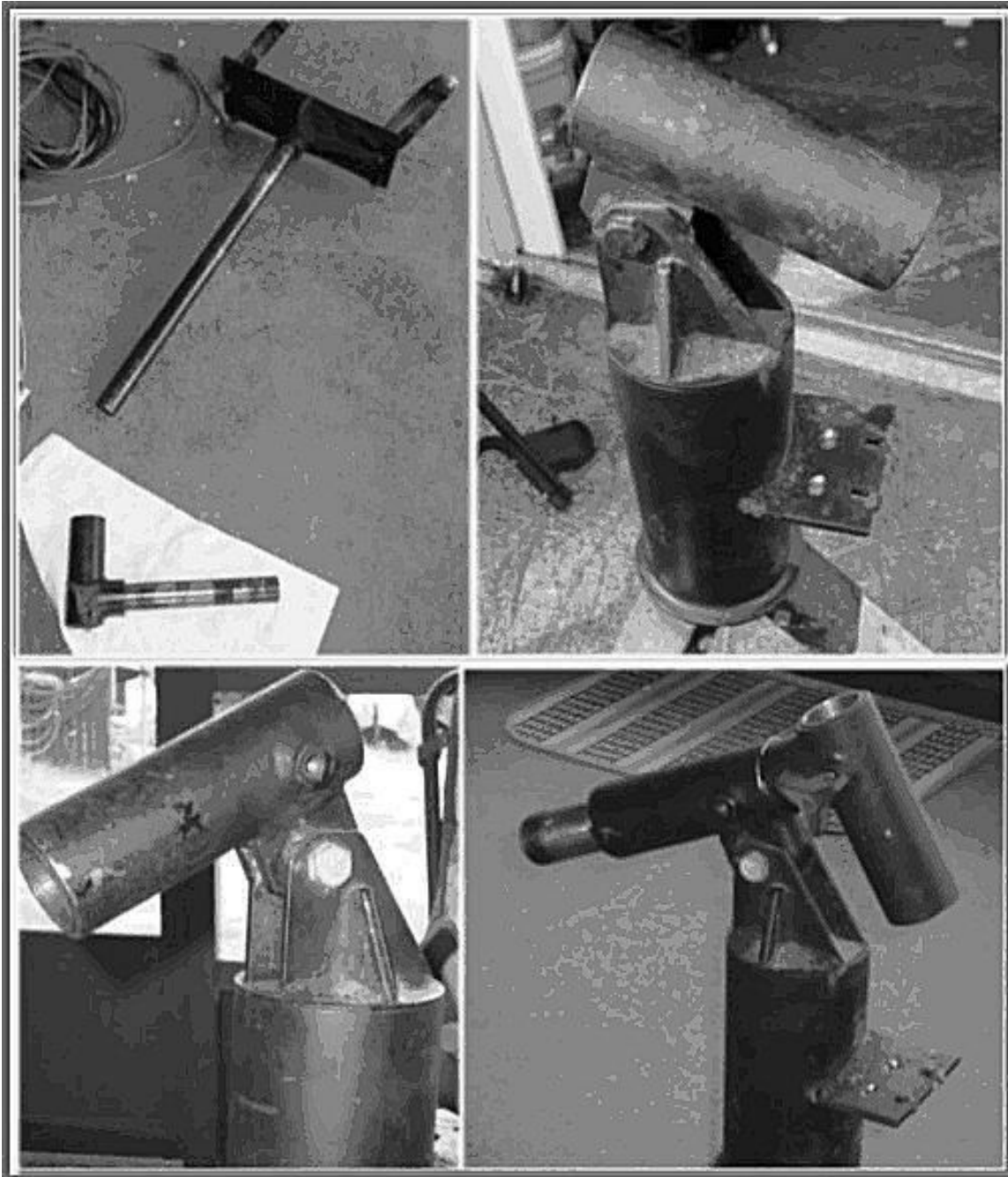
TOP-LEFT: Rust removal from shafts and cleanup. TOP-RIGHT: Polar housing and pier with both shafts removed. BOTTOM-LEFT: Polar housing reversed and attached to pier hub with new bolt and nut. BOTTOM-RIGHT: Bearings and shafts cleaned and polar shaft installed in housing.
