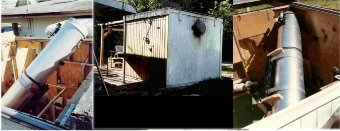
Figure 1. Pre-hurricane Andrew photos of roll-off roof observatory and 12.5" f/7 Newtonian telescope. A bit cramped, but this was a cozy and productive setup for many years. 1-5/8th inch Chain-link fence rail system for the roll-off-roof observatory shown in left and right images.
