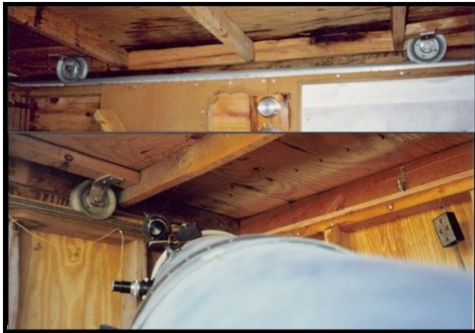
Figure 2. Photos the casters on a chain-link fence rail system in my roll-off-roof observatory. Rail is 1.625 inch diameter chain-link top rail.
